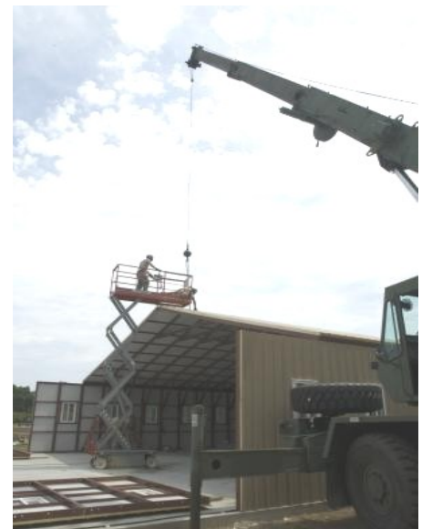
Spc. Verrek E. Green & Cpl. Christopher T. Tibbs from the 390th Engineer Company, unhook a crane from the roof while constructing the 100-person classroom.
